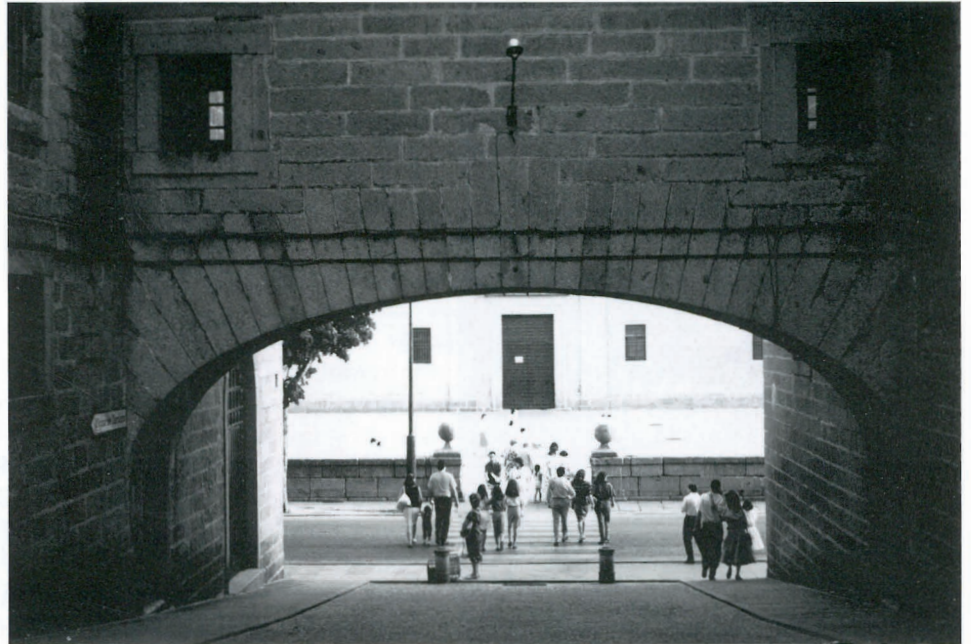
22. Bridge connecting two north service buildings ( Casas de Oficios ) at the Escorial, designed by Juan de Herrera, c.1585; restored by Juan de Villanueva, c.1785.
